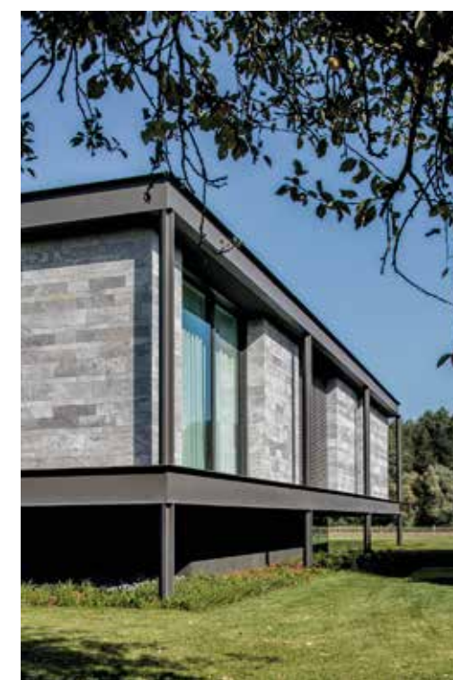
pierre de varenne - donsato architecture by CAAN architecten – Gent photography Thomas De Bruyne
